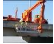
UNDER BRIDGE CONDUIT CONSTRUCTION SUPPORT
