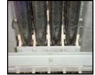
BRIDGE ATTACHMENT HANGERS & SUPPORTS
